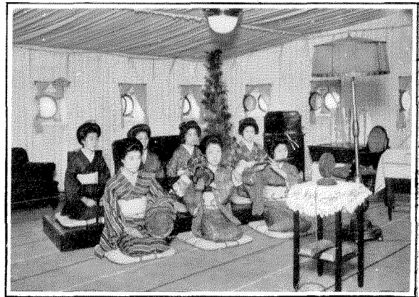
Osaka Broadcasting Station—Japanese musicians in studio of temporary station
