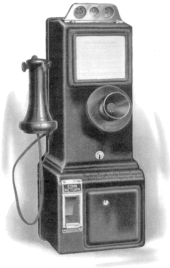
Figure 9—No. 50-G. Multi-Coin Pre-payment Collector Arranged for Manual Service
