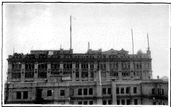
Osaka Broadcasting Station—Temporary installation of W.E. Type No. 101-B equipment on the roof of the Mitsukoshi Department Store Reception of this station has been reported from Pennsylvania—(October 25, 1926)
