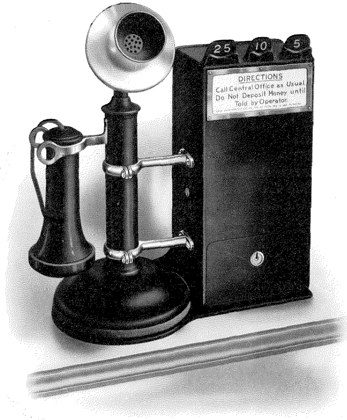
Figure 5—Post-Payment Multi-Coin Collector and Desk Stand Rigidly Mounted
